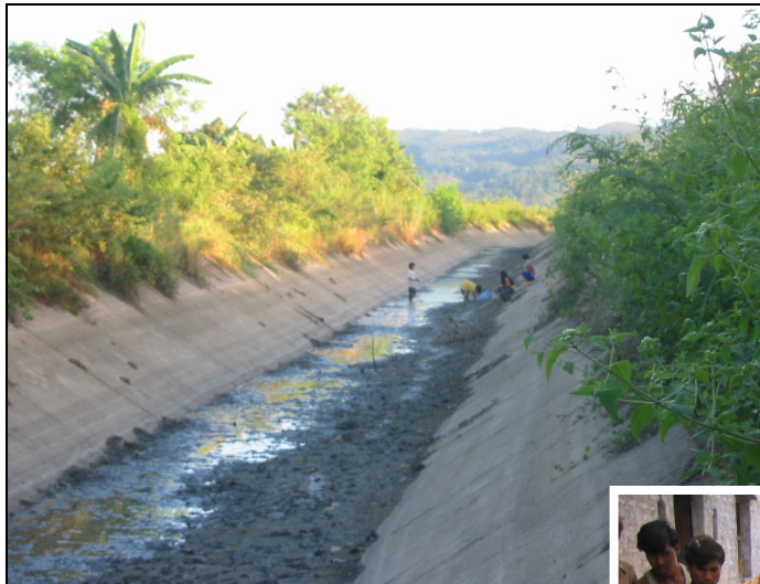
Empty main canal of the Bohor Irrigation Project, the Philippines
