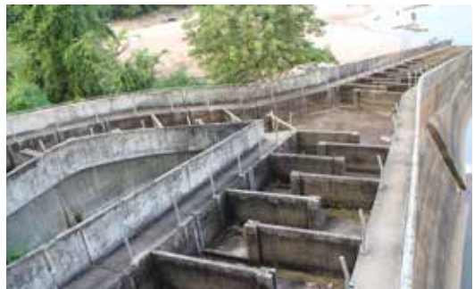
Fish Ladder at the Pak Mun Dam
