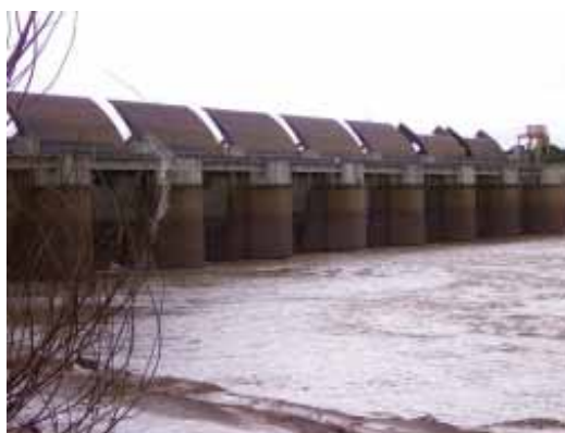
Pak Mun Dam
