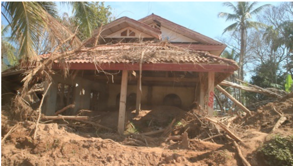
House damaged in disaster (photo taken in Dec. 2018)
