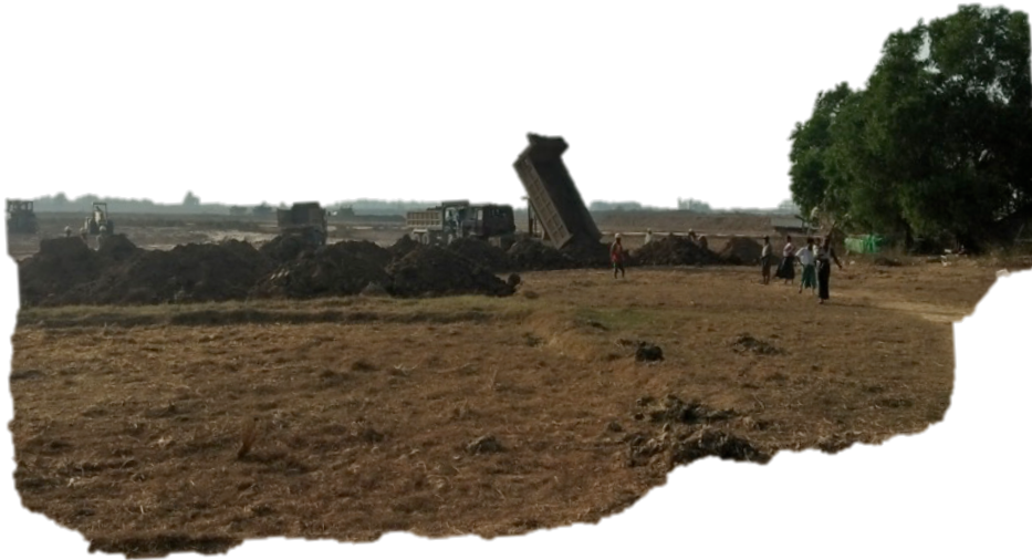
Photo: Relocation district as construction proceeds (taken in February 2020)
