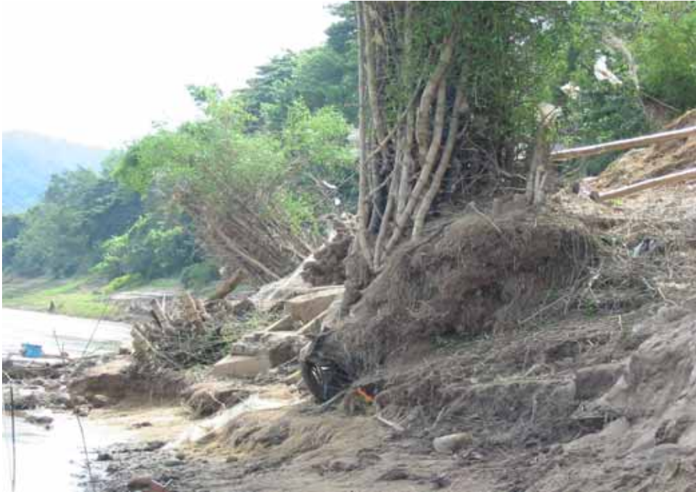
Extraordinary water fluctuation of the Mekong River is believed to be the cause of bank erosion at villages in Chiang Khong, November 2004,
